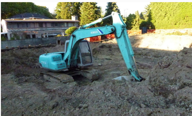
Pictured: Construction underway
